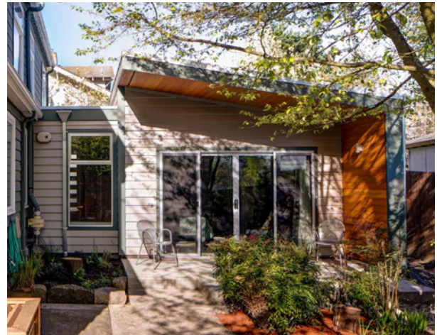
An attached ADU with screening to provide privacy from neighboring buildings. Photo courtesy Hammer and Hand.
