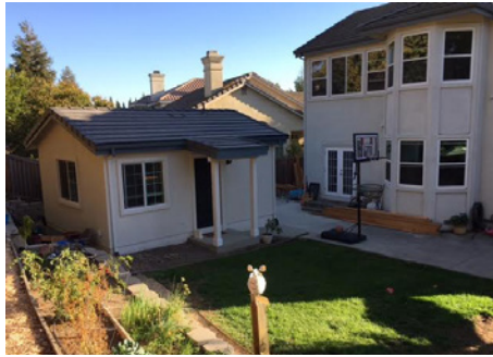
A detached ADU and a two-story primary dwelling. Photo Courtesy The Small House Catalogue
